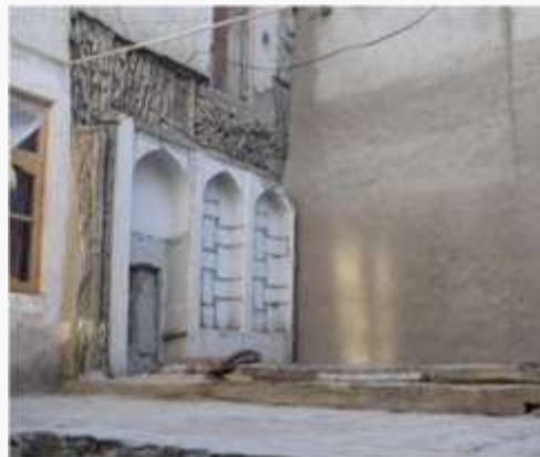
5-picture. As a result of the demolition of the room, the window was filled with corundum.
